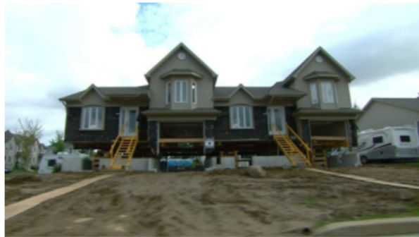
This house is one of hundreds that have undergone repairs to fix damage caused by pyrrhotite.
